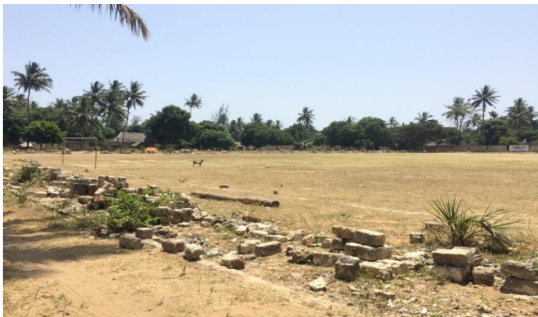
Figure 2 The unfinished and abandoned football stadium in Tiwi
